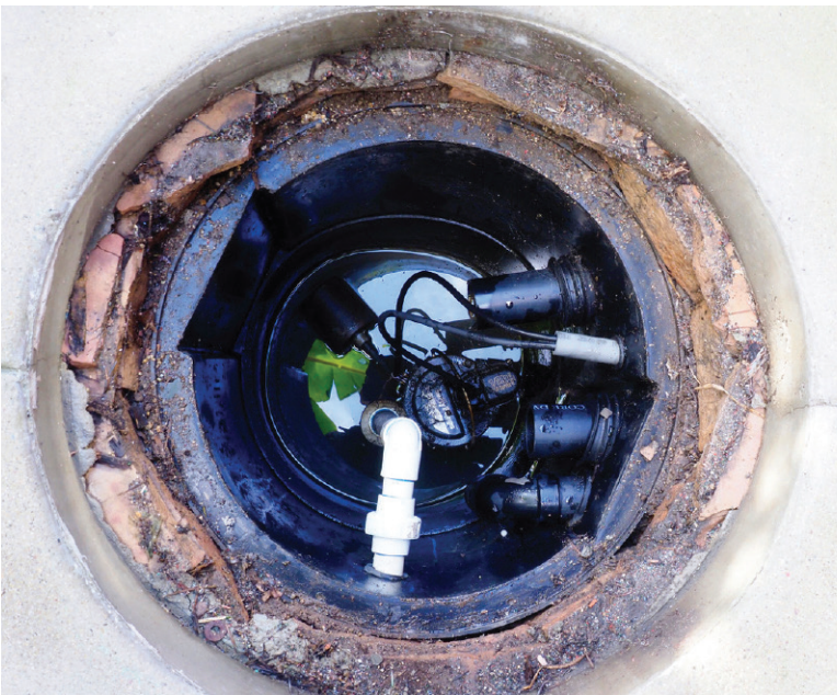
Our greywater system surge tank and pump.
